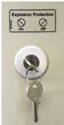
Figure 4.8 Control box key switch
